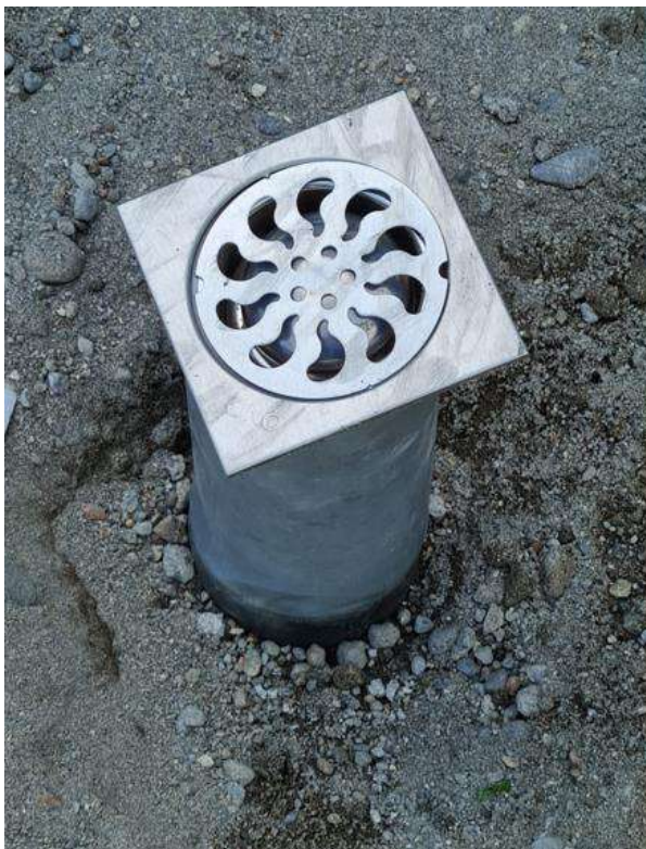
Penambahan lubang biopore diantara paving blok.
